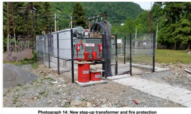
Photograph 14: New step-up transformer and fire protection
