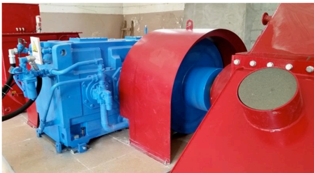
Photograph 4: Power unit - generator
